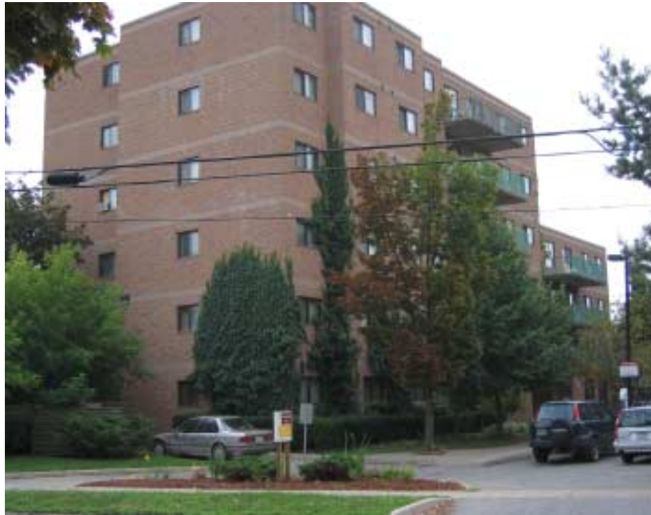
Bethlehem Place's current transitional apartment building.
